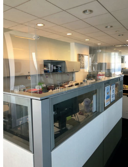
Protective Barriers for Cubicles
